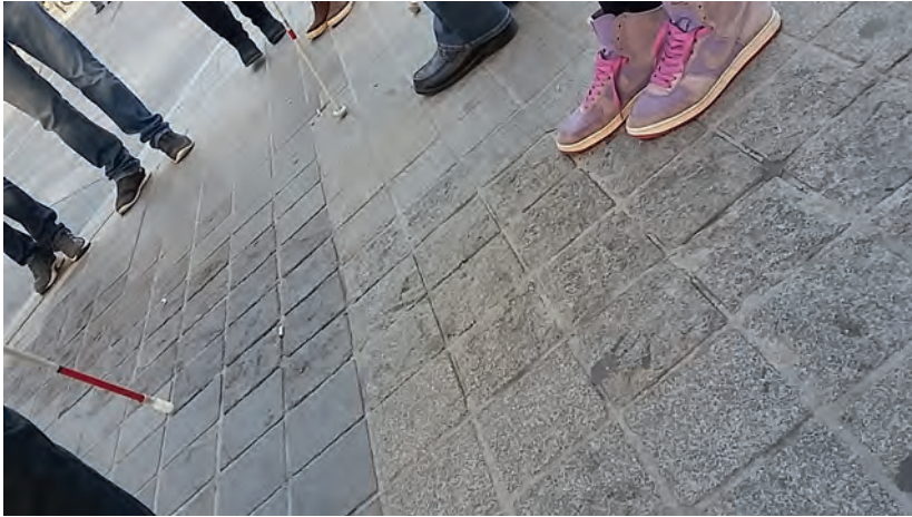
Figure 1 BBSB members testing the ‘creative’ approach to the podotactile pavement: a series of granite tiles with irregular, mountain-like shapes
