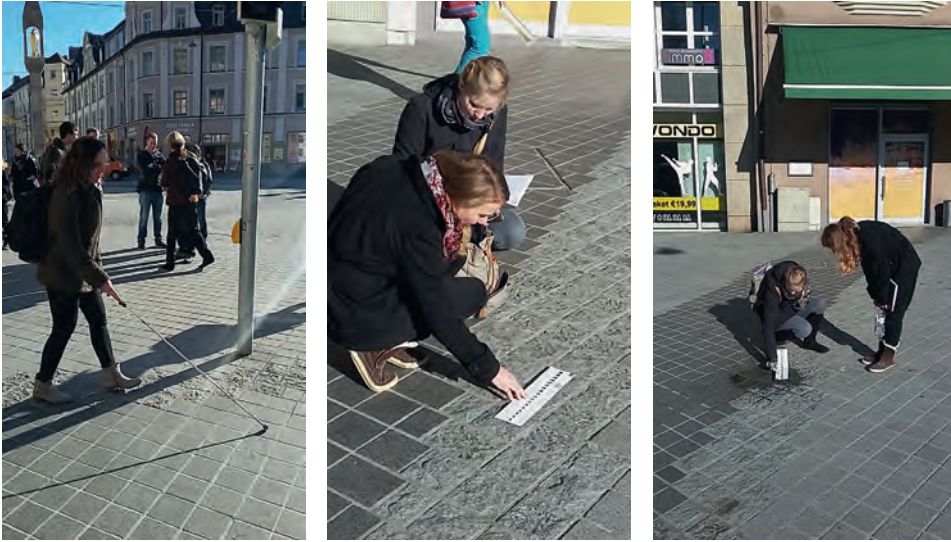
Figures 3–5 The BBSB delegation tests different aspects of Pasing’s Marienplatz new shared street. Left: Detail of the dropped-kerb bike lane. Centre: Dropped-kerb bike lane running through the sidewalk. Right: An older person crosses over the dropped-kerb bike lane and car lane without difficulties
