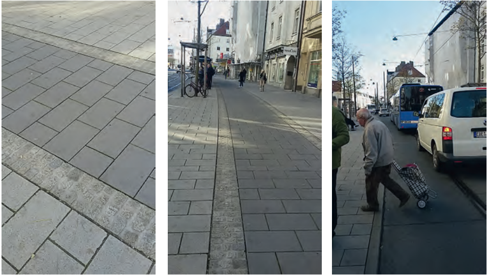
Figures 6–8 The BBSB delegation tests different aspects of Pasing’s Marienplatz new shared street. Left: Melanie Egerer tests the tactile differentiation of the podotactile pavement. Centre and Right: BBSB interns use different tools to test the colour contrast between the podotactile pavement and the regular pavement
